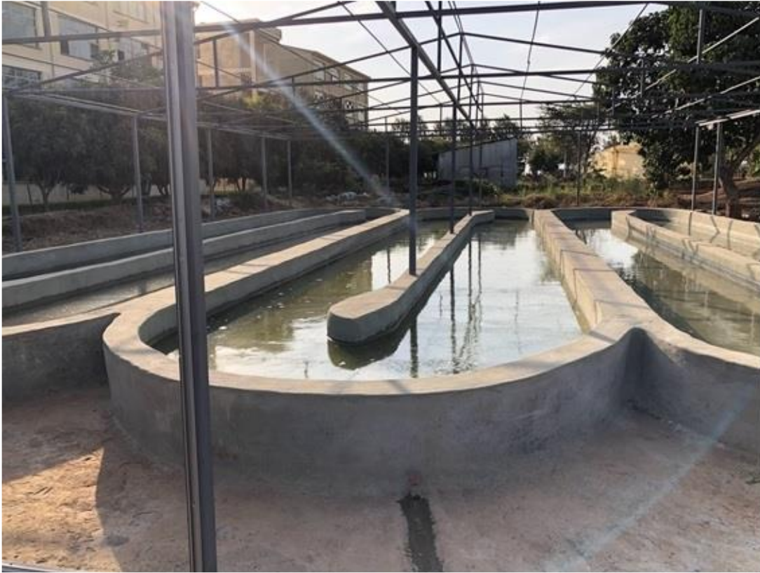
Fig. IV-2. Raceway ponds constructed by the SATREPS EARTH project at Bahir Dar University, Ethiopia, for the large-scale cultivation of microalgae.
